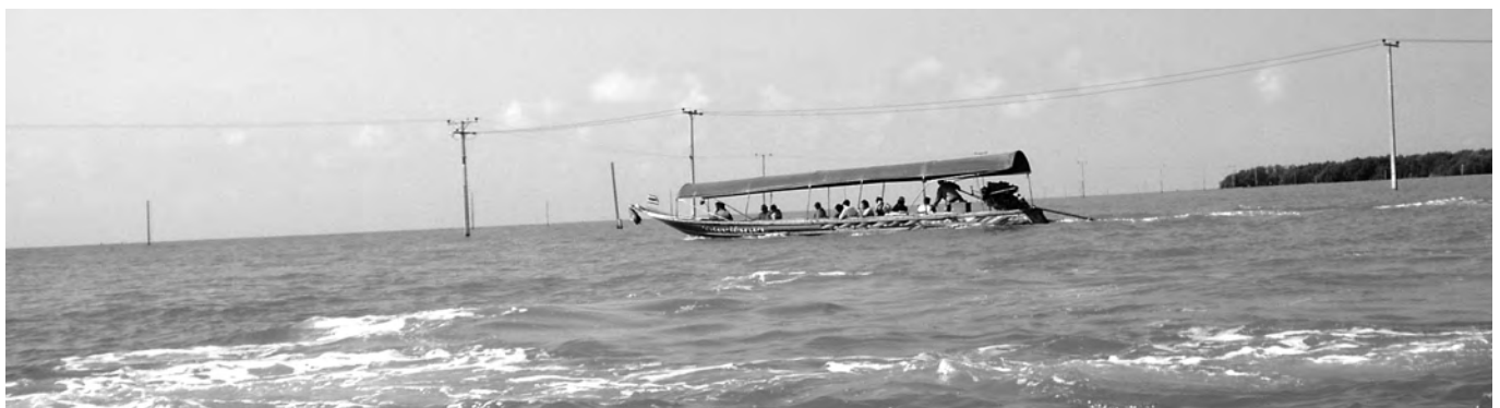
Figure 6 A line of telegraph poles south of Bangkok: built on subsiding land, they are now as much as a kilometre out to sea.
